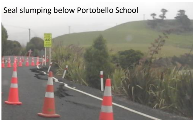
Water gouges out the edge of the road
