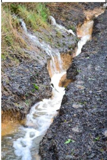
Water gouges out the edge of the road
